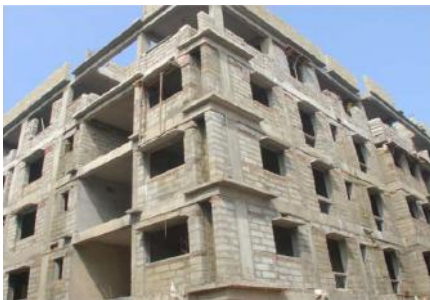
WATER CURING IS NOT REQUIRED
